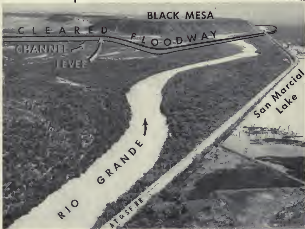
REROUTING THE RIO —The channel for the Rio Grande, dug through the 30-mile-long swamp, is shown above, as solid line. A levee (solid black line) the channel and meso will for way" or "paddock" for the runs wild and washes out the dike on the right side of the the left of old Fort Croig is shown temporary levee and emergency to take care of spring runoff. The four emergency ditches during summer and fall by the State, servancy District are also shown dashed lines. At left, an aerial the 2-mile-wide river flood plain the inundated town of San flooded in 1929. Map above by Region 5, at right by Graphic Washington, D. C.
